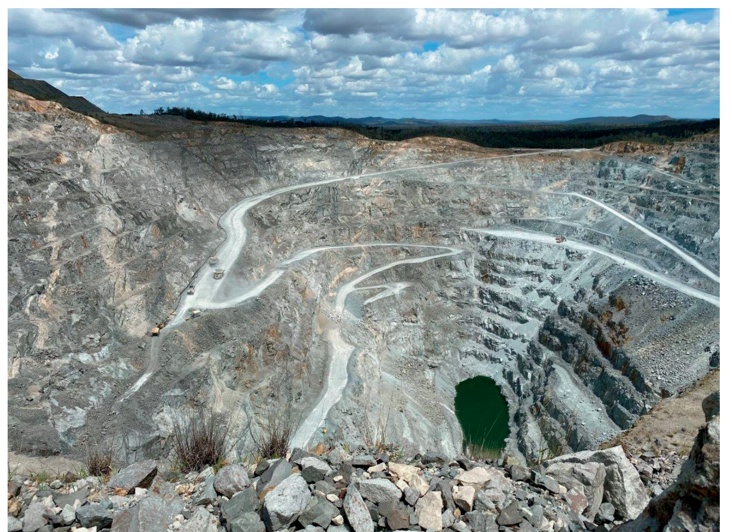
Mt Rawdon mine pit (proposed lower reservoir location).
