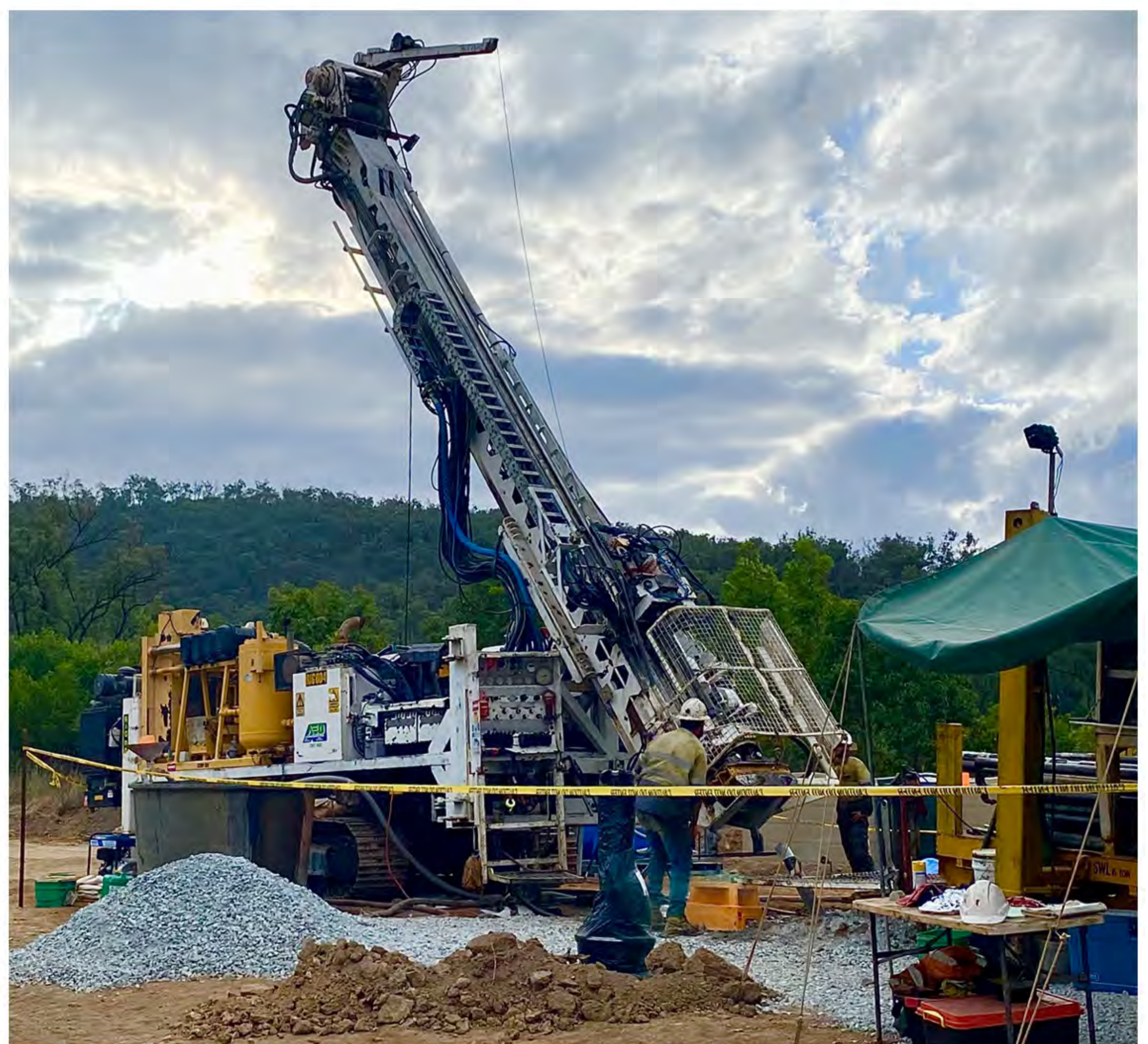
Geotechnical drilling rig
