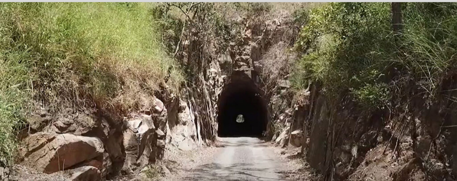
The heritage listed Boolboonda Tunnel in Mount Perry (Photo by Bundaberg Now)
